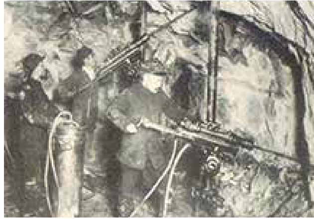
Drilling with imported rock drills
