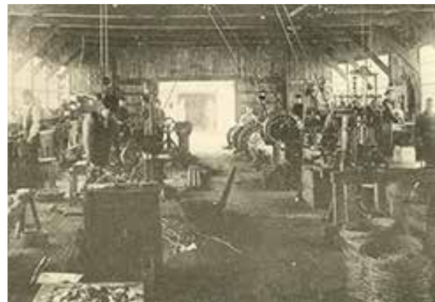
Ashio Electric Machinery Repair Works
