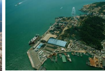
Hibi Joint Smelter
