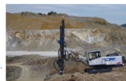
Hydraulic crawler drills
