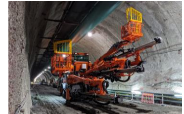
Tunnel drill jumbos
