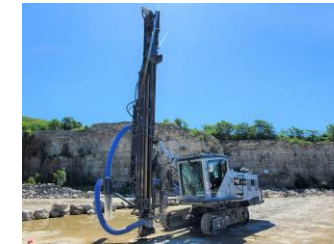
Hydraulic crawler drills
