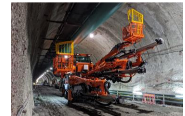
Tunnel drill jumbos
