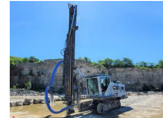
Hydraulic crawler drills
