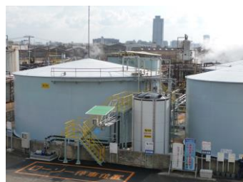
Manufacturing plant of sulfuric acid
