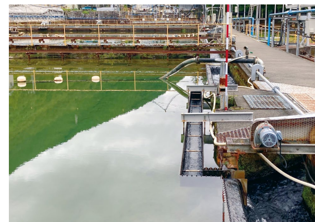
Settlement pond overflow weir extension (Nakasai water purification plant)
