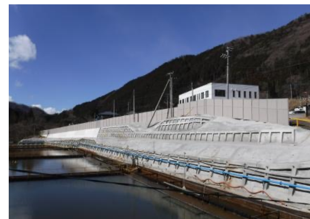
Stone retaining wall reinforcement: Stage III (Nakasai water purification plant)
