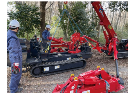
Disassembled crane Assembling in mountainous area
