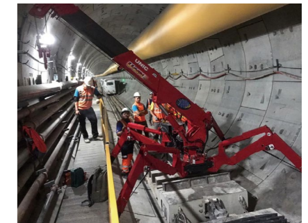
Battery-powered crane Crane operation in tunnel
