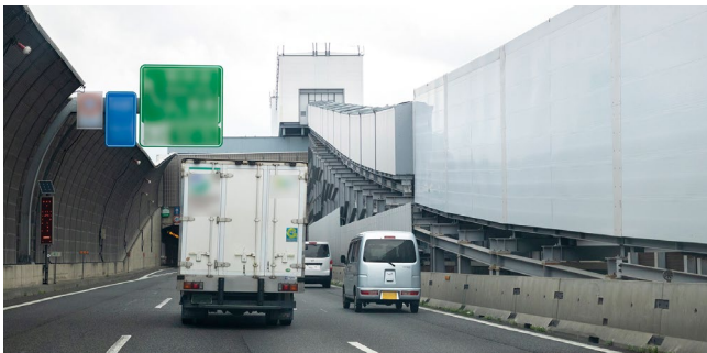
Construction of an expressway tunnel Long-distance, high-capacity, curved-belt conveyor
