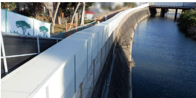
Construction of a control pond SICON® enclosed hanging belt conveyor
