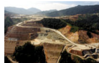
Copper and gold mine, Batu Hijau Mine (Indonesia) in which Furukawa Co., Ltd. invests
