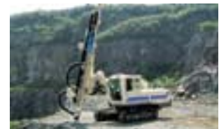
Hydraulic crawler drills
