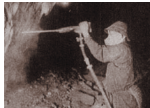
The first domestic rock drill was developed at Ashio.
