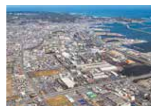
Onahama Smelting and Refining Co., Ltd.
