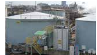
Sulfuric acid production plant
