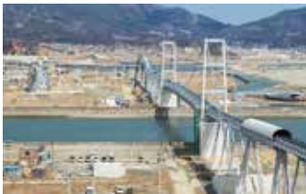
Project for relocating people to higher ground in Rikuzentakata City (installation completed in fiscal 2015, demolition in fiscal 2017)
