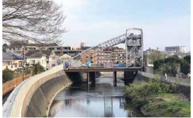
Enclosed hanging belt conveyor provided to the Sakaigawa-Kanamori retention basin project (Machida City, Tokyo)
