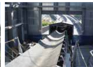
Belt conveyor installation work (Tokyo Gaikan Expressway)
