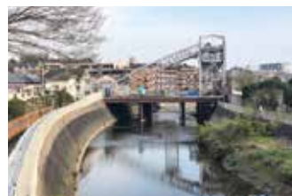
Belt conveyor installation work (Sakaigawa-Kanamori retention basin project)
