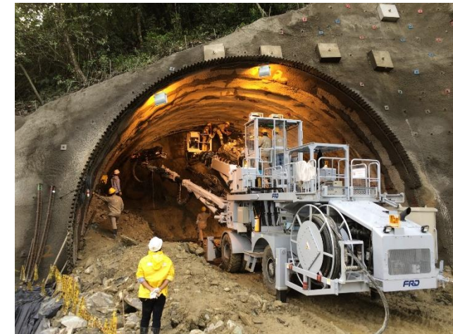
Drill Jumbo in operation at overseas tunnel excavation site
