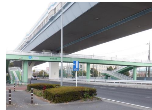
Route 17 Shin-omiya Bypass pedestrian bridge. One of the bridge constructions that were awarded for Excellent Safety Management Order Winner Award.
