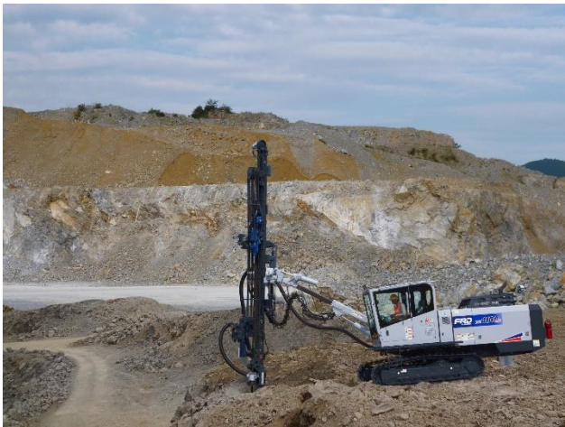
Hydraulic Crawler Drill in operation at overseas quarry site
