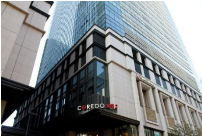
Muromachi Furukawa Mitsui Building (commercial name: COREDO Muromachi 2) Nihonbashi Muromachi, Chuo-ku
