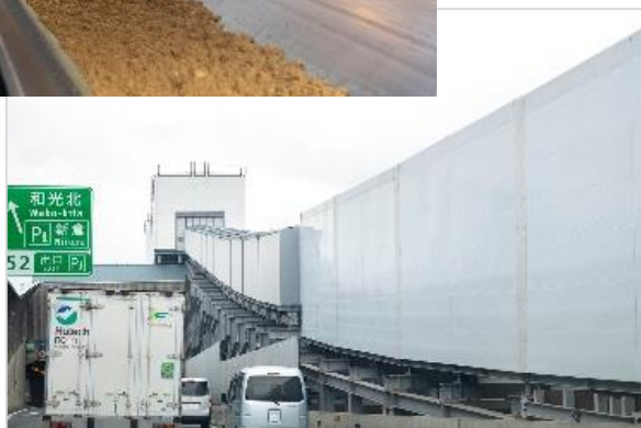
Belt Conveyors designed for the Tokyo Outer Ring Road project
