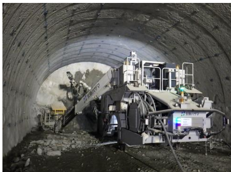
Tunnel drill jumbo using remote technology. (Jointly developed with HAZAMA ANDO CORPORATION and MAC.)
