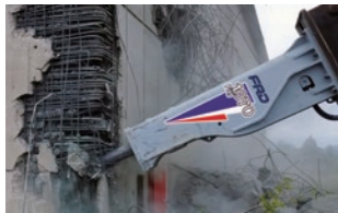
Hydraulic breakers These machines are used to break rocks and crush concrete.
