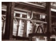
The Furukawa / Outokumpu flash smelting plant
