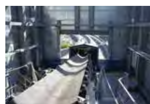
Belt conveyor installation work (Tokyo Gaikan Expressway)
