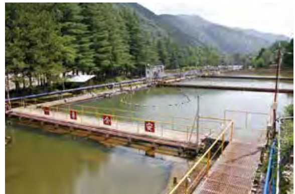
The Nakasai Water Treatment Plant operates 24 hours a day.
