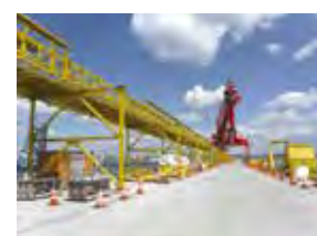
Belt conveyor installation work (Onahama)
