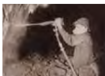
The first domestic rock drill was developed (for the Ashio Copper Mine).
